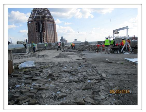
Next we repeated the same process to **remove the 2" extruded polystyrene insulation board**. We had to be careful as we did not want to disturb the coal tar pitch. The design called for only removing unattached areas and leaving as much of it in place so as to not create a situation
