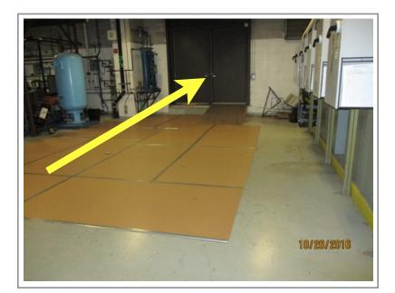
Next we repeated the same process to **remove the 2**" **extruded polystyrene insulation board**. We then removed extensive areas of lose coal tar pitch and conducted repairs to the barrier. Some of the removal work was challenging due to not just the **multiple elevations** but also the tight areas in the cooling tower area with **clearance enough only to crawl**.
