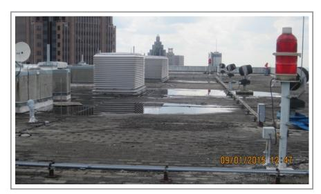
foam. The top is a fully adhered 60 mil TPO membrane. This also meets the current R value per building code, that has changed considerably since the 1980s when the building was constructed. Additionally this allowed us to secure a 20 year, no dollar limit warranty.
