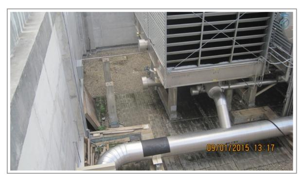
We recommend the installation of 2,000 sf of walk pads in the area of the roof where the mechanical equipment is located. This protected the roof system and allow for the servicing of the extensive equipment.
